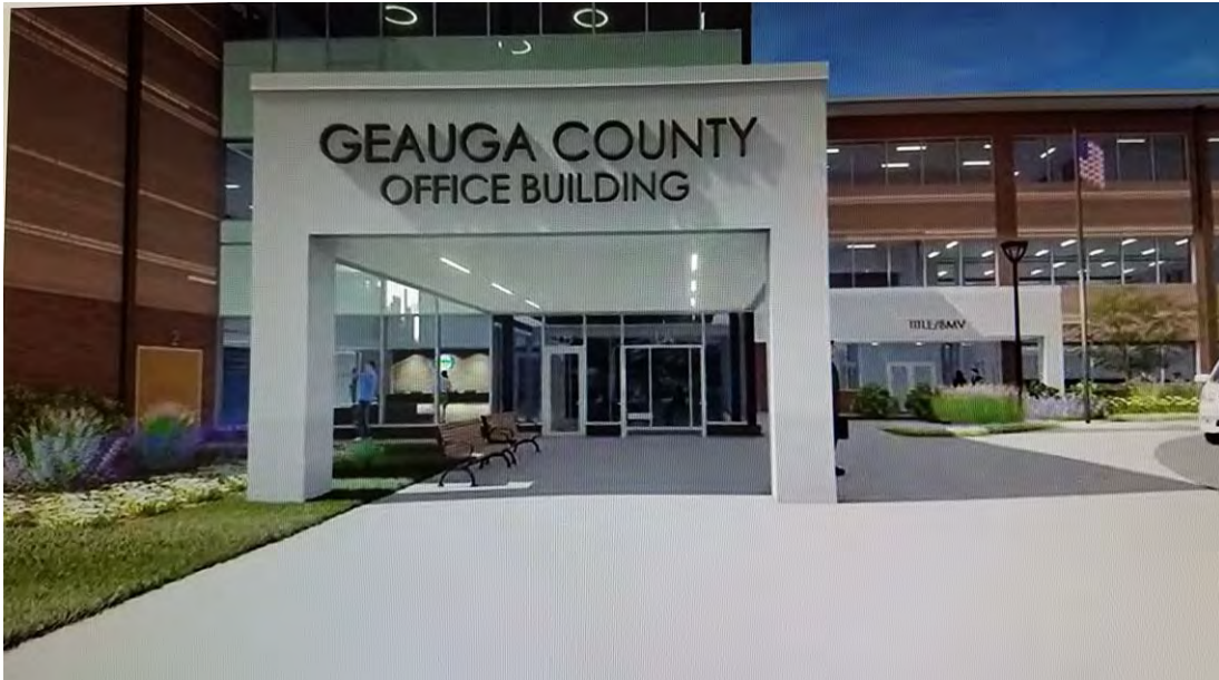
Main entrance and lobby
